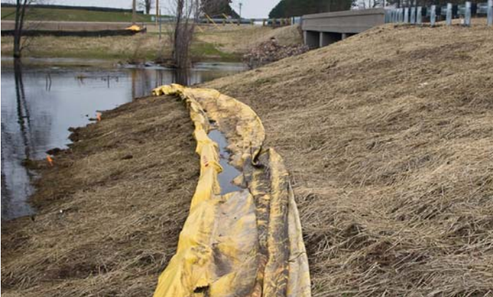
Lay out materials to dry.
